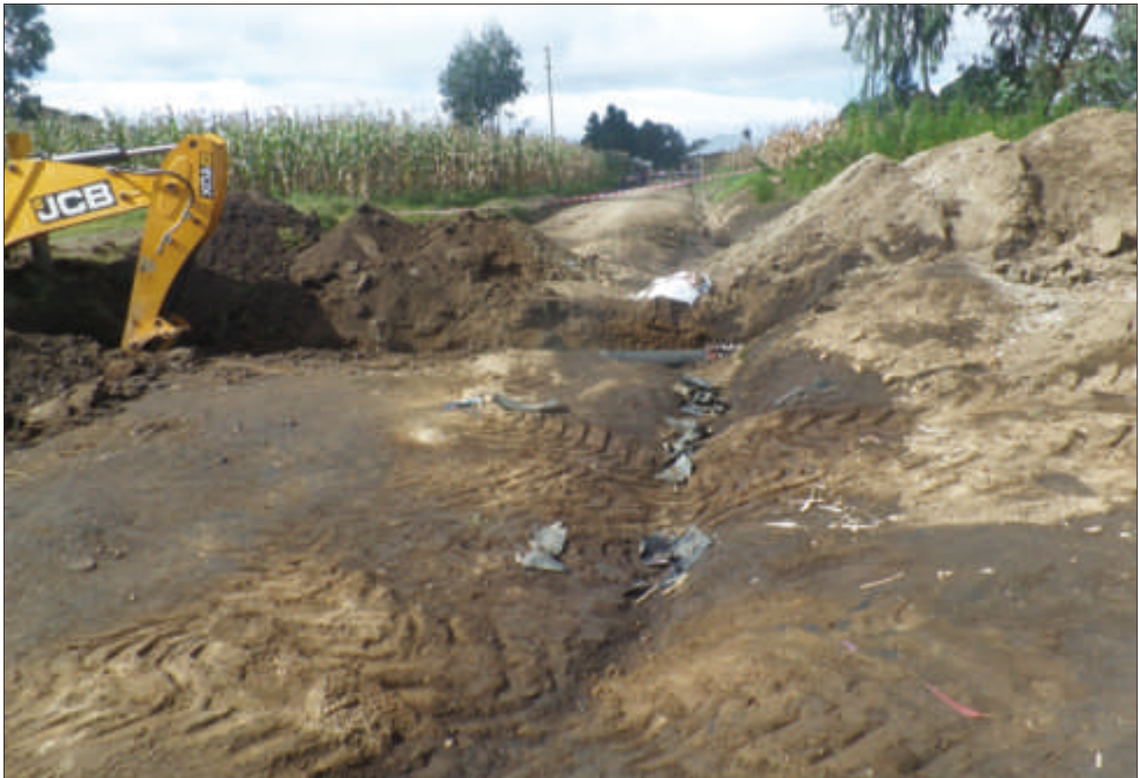
Figure 32: The pipeline's road-crossing where the TARURA contractor was undertaking excavation for the construction of a road and eventually damaged the pipeline. The part of the land was polluted with spilt diesel.
