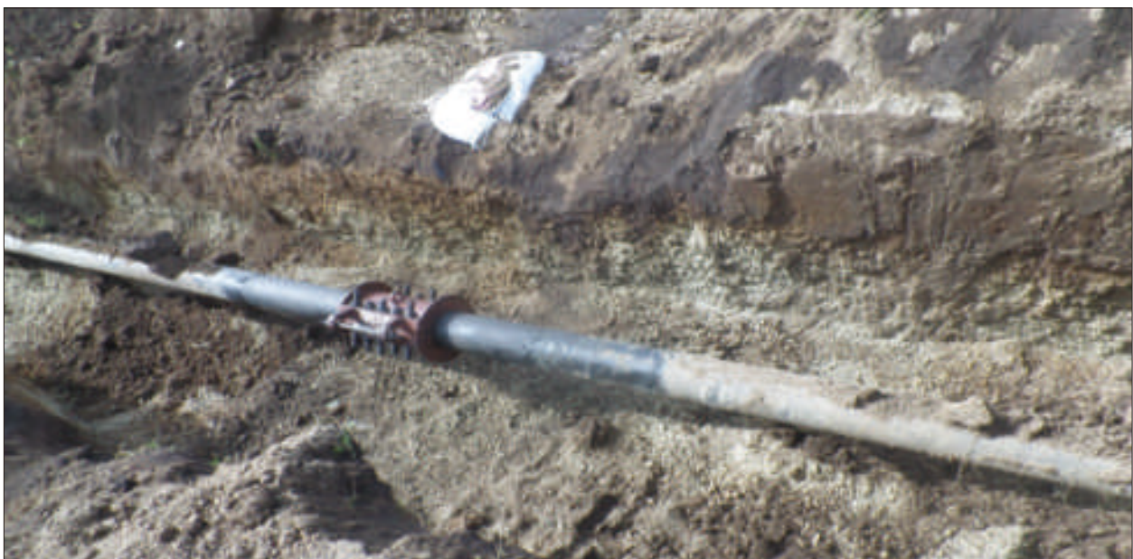
Figure 33: The damaged part of the pipeline was temporarily fixed before connecting the pipeline with the spool piece of the pipe.
